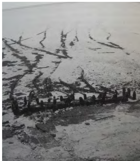
PLUTO arrived on the Island from Hampshire at Thorness Bay, and the remnants can still be seen on a low tide.
