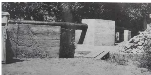
A raised section of the Pluto pipeline at Shanklin. Part of the pipe can still be seen in Shanklin Chine.
